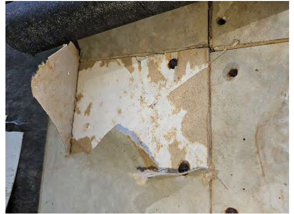
Photo 5.4: Water damaged gypsum sheathing, paper facing, and fasteners.
