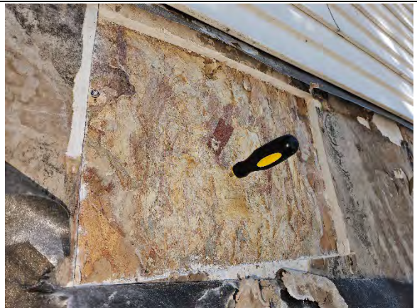
Photo 4.10: Water damaged OSB sheathing.
