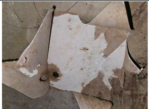
Photo 5.6: Water damaged gypsum sheathing, paper facing, fasteners, and core.
