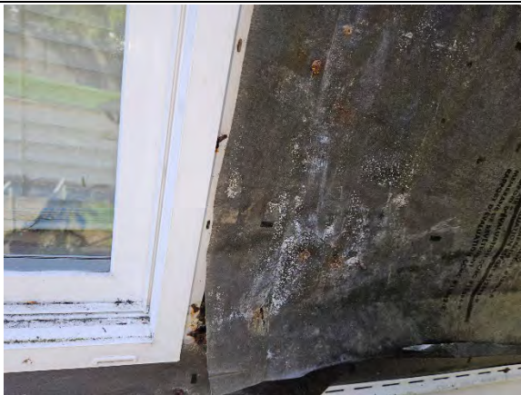
Photo 16.3: Water damaged WRB.
