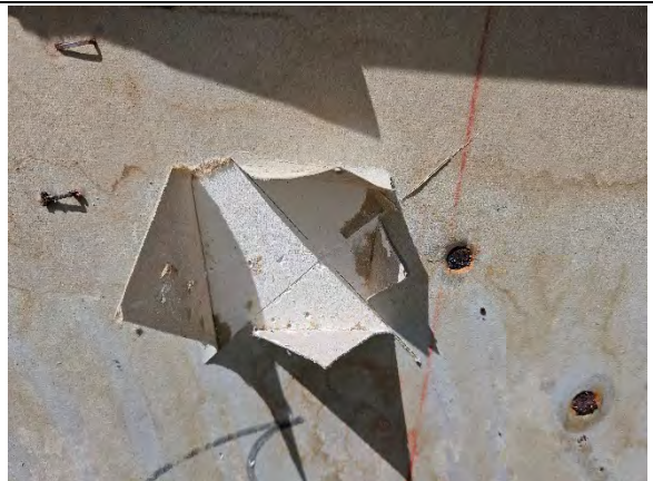
Photo 13.6: Water damaged gypsum sheathing, paper facing, and fasteners.
