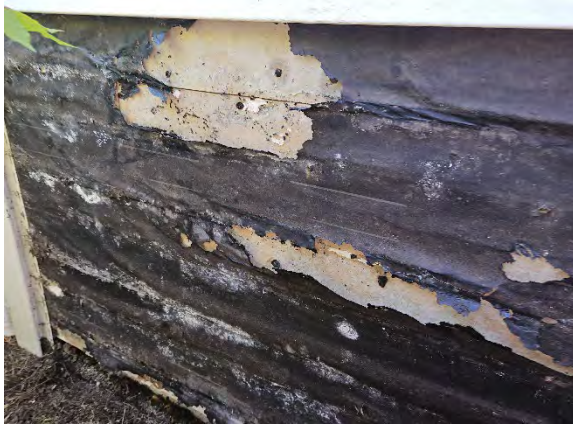
Photo 8.3: Water damaged WRB.
