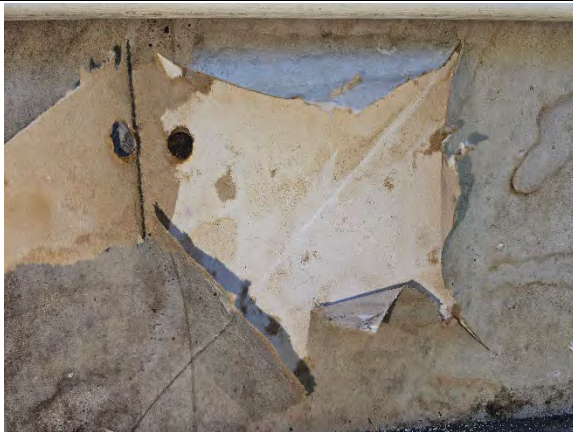
Photo 15.5: Water damaged gypsum sheathing, paper facing, and fasteners.
