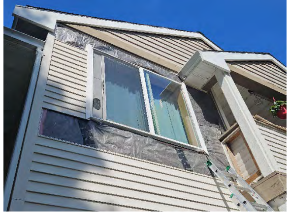
Photo 13.2: Opening following cladding removal.
