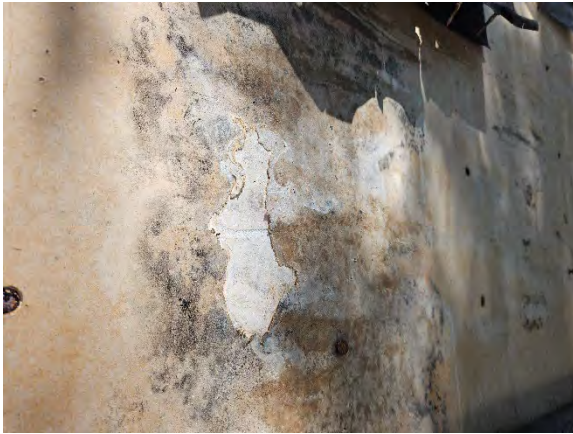
Photo 4.7: Water damaged gypsum sheathing, paper facing, fasteners, and core.
