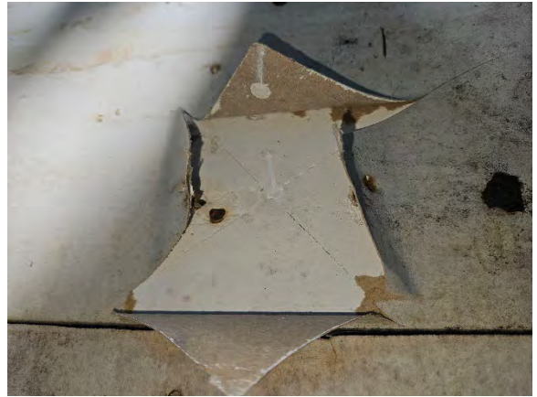
Photo 3.8: Water damaged gypsum sheathing, paper facing, and fasteners.
