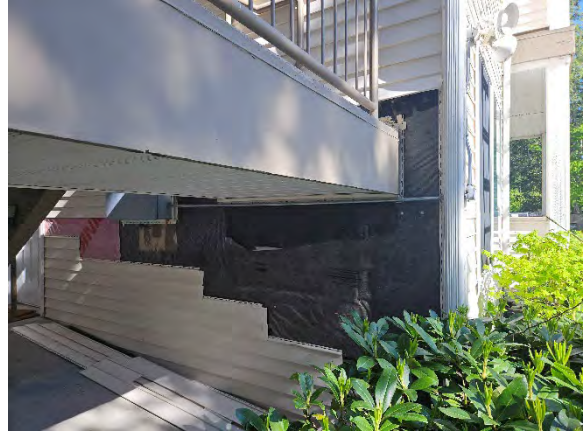
Photo 12.2: Opening following cladding removal.
