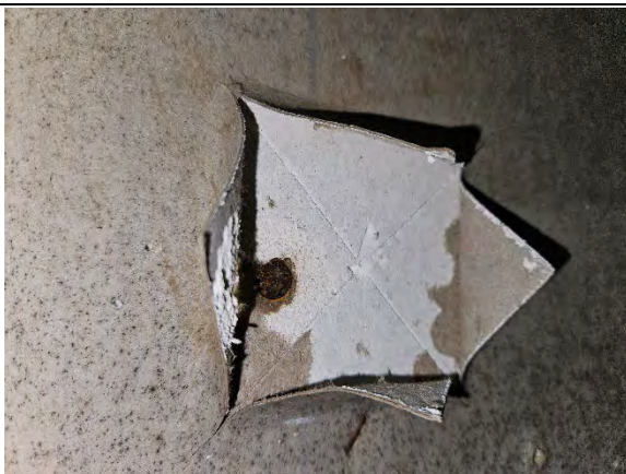
Photo 2.5: Water damaged gypsum sheathing, paper facing, fasteners, and core.
