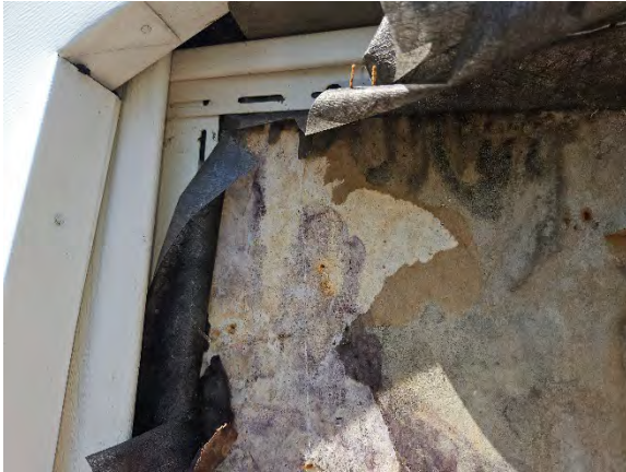
Photo 13.3: Water damaged gypsum sheathing, paper facing, fasteners, and core.
