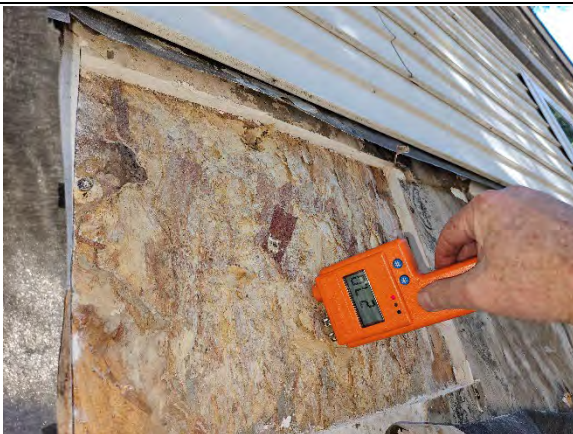
Photo 4.11: Wet reading (27.0) at OSB sheathing.
