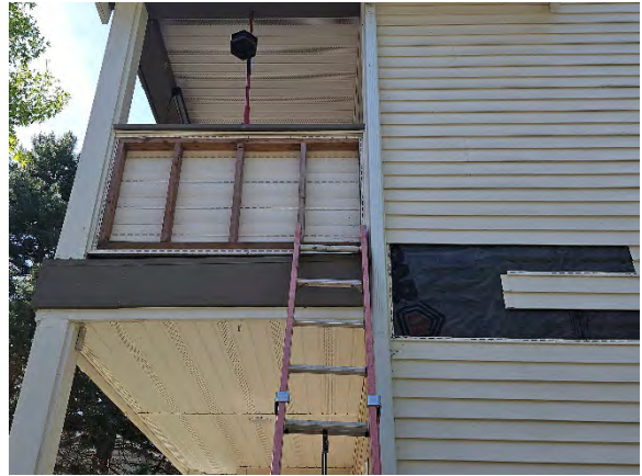
Photo 15.2: Opening following cladding removal.
