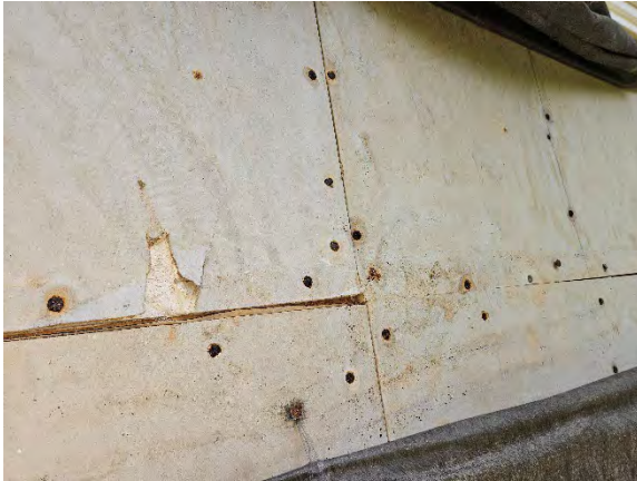
Photo 14.3: Water damaged gypsum sheathing, paper facing, fasteners, and core.
