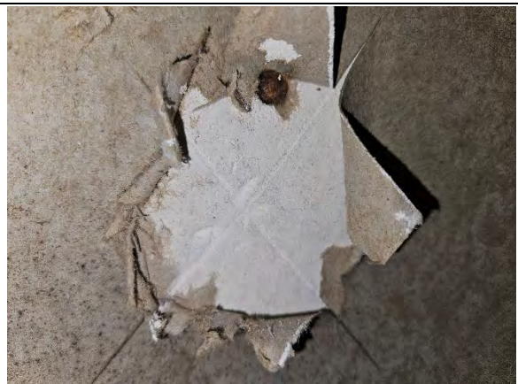
Photo 2.6: Water damaged gypsum sheathing, paper facing, and fasteners.
