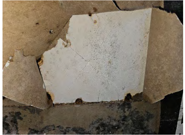
Photo 12.4: Water damaged gypsum sheathing, paper facing, fasteners, and core.
