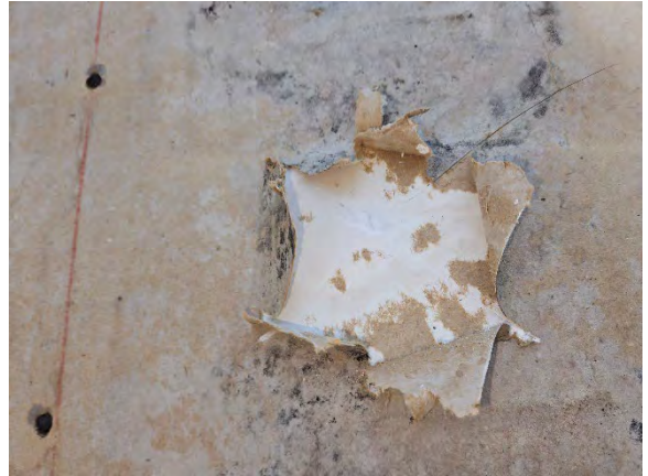
Photo 4.4: Water damaged gypsum sheathing, paper facing, and fasteners.
