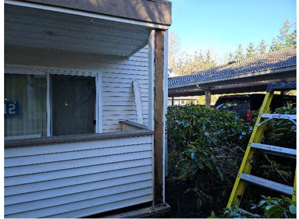
Photo 2.2: Opening following cladding removal.
