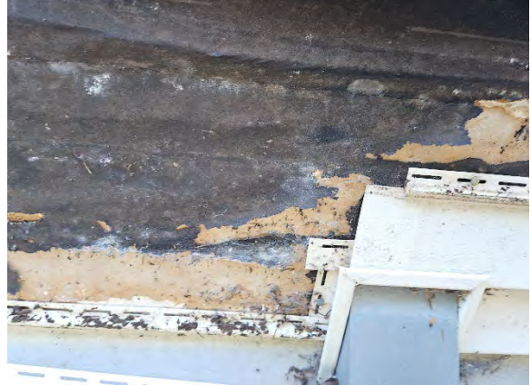
Photo 8.4: Water damaged WRB.
