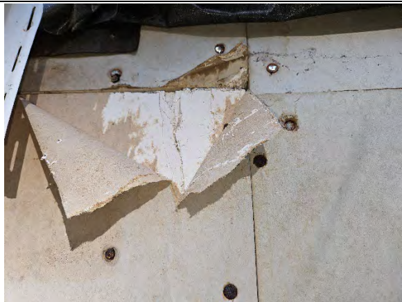
Photo 5.5: Water damaged gypsum sheathing, paper facing, fasteners, and core.
