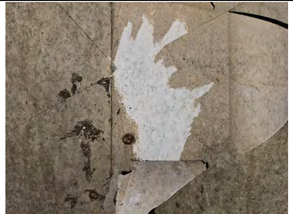
Photo 3.4: Water damaged gypsum sheathing, paper facing, and fasteners.
