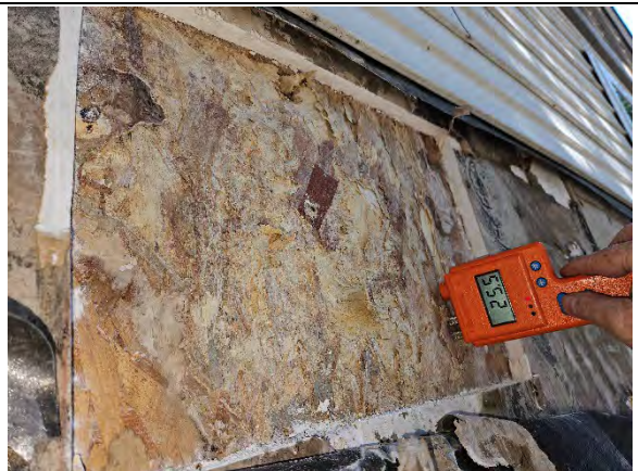
Photo 4.12: Wet reading (25.5) at OSB sheathing.
