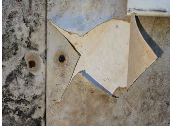
Photo 15.4: Water damaged gypsum sheathing, paper facing, and fasteners.
