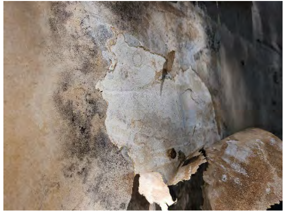
Photo 4.8: Water damaged gypsum sheathing, paper facing, fasteners, and core.
