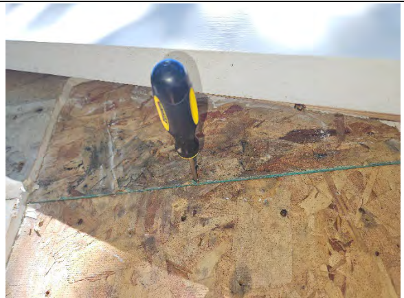
Photo 3.10: Water damaged OSB sheathing.
