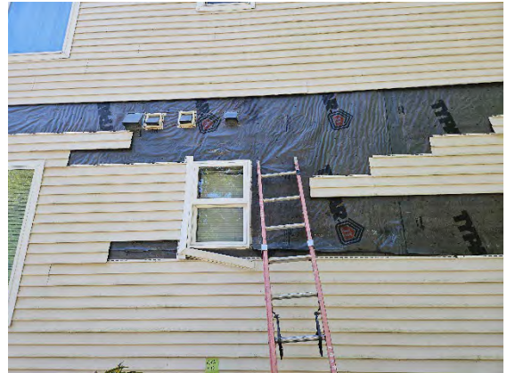
Photo 16.2: Opening following cladding removal.
