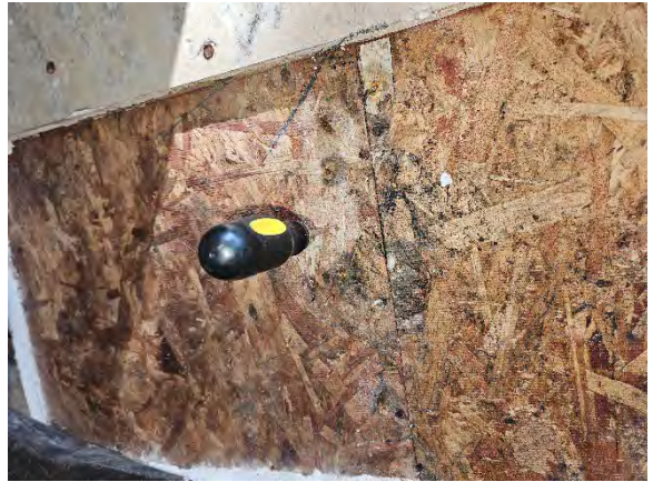
Photo 12.8: Water damaged OSB sheathing.
