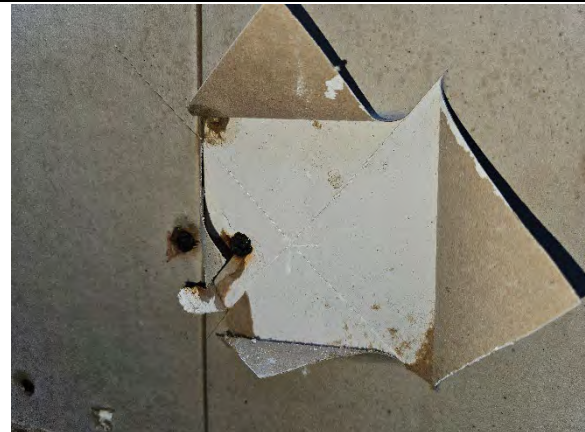
Photo 1.6: Water damaged gypsum sheathing, paper facing, and fasteners.
