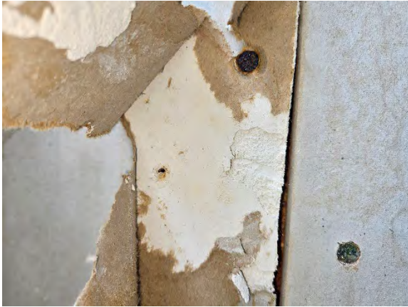
Photo 11.3: Water damaged gypsum sheathing, paper facing, fasteners, and core.
