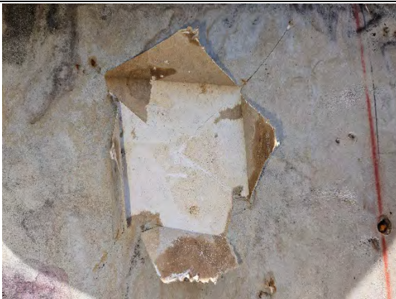
Photo 13.5: Water damaged gypsum sheathing, paper facing, and fasteners.
