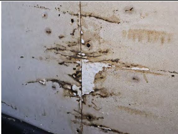
Photo 1.5: Water damaged gypsum sheathing, paper facing, fasteners, and core.
