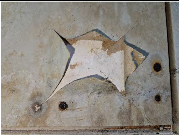
Photo 14.5: Water damaged gypsum sheathing, paper facing, and fasteners.
