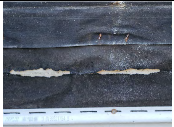
Photo 1.4: Water damaged WRB.
