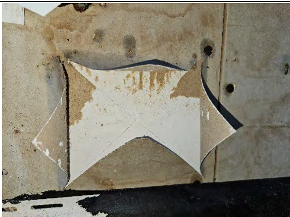
Photo 1.5: Water damaged gypsum sheathing, paper facing, and fasteners.
