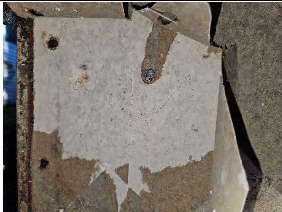
Photo 3.3: Water damaged gypsum sheathing, paper facing, and fasteners.
