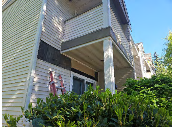
Photo 11.2: Opening following cladding/soffit removal.
