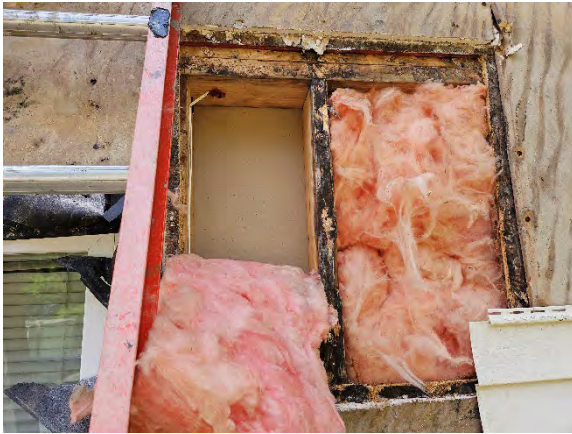
Photo 16.13: Water damaged framing.
