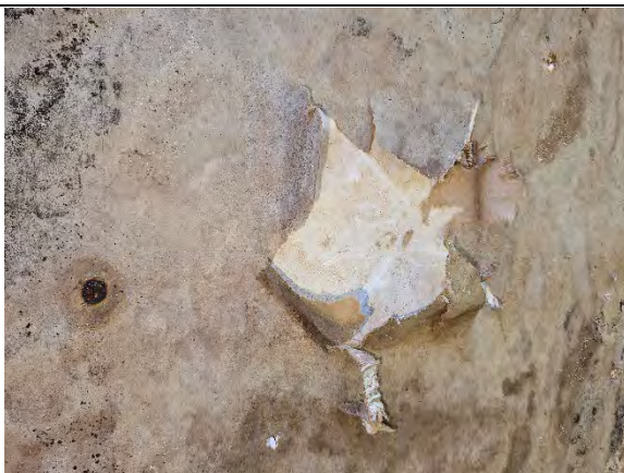
Photo 16.5: Water damaged gypsum sheathing, paper facing, and fasteners.
