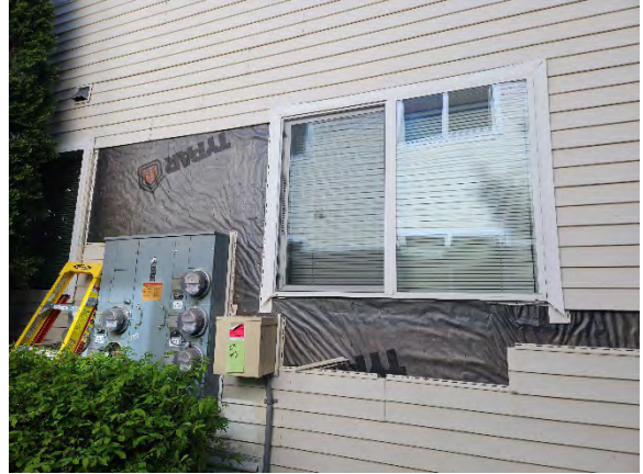
Photo 6.2: Opening following cladding removal.
