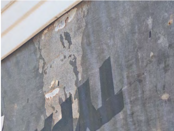
Photo 4.3: Water damaged WRB.
