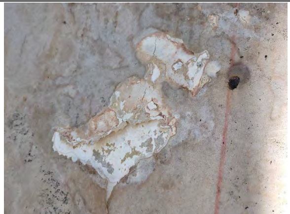
Photo 4.6: Water damaged gypsum sheathing, paper facing, fasteners, and core.
