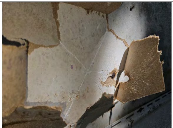
Photo 3.6: Water damaged gypsum sheathing, paper facing, and fasteners.
