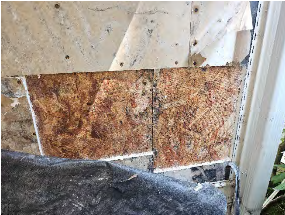
Photo 12.7: Water damaged OSB sheathing.
