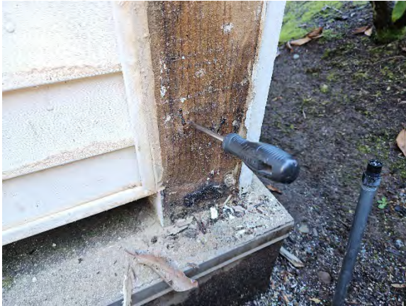
Photo 2.3: Water damaged deck column.
