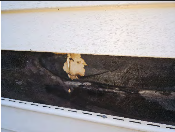
Photo 1.3: Water damaged WRB.
