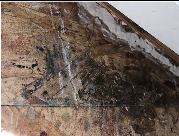
Photo 3.9: Water damaged OSB sheathing.
