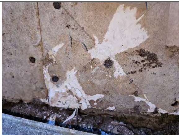
Photo 3.5: Water damaged gypsum sheathing, paper facing, fasteners, and core.
