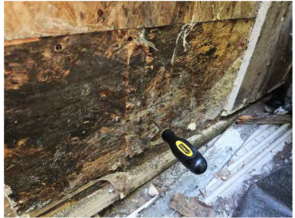
Photo 5.8: Water damaged OSB sheathing.
