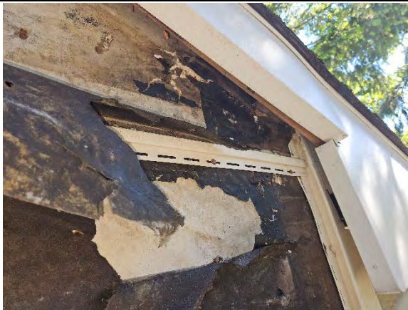
Photo 3.3: Water damaged WRB.
