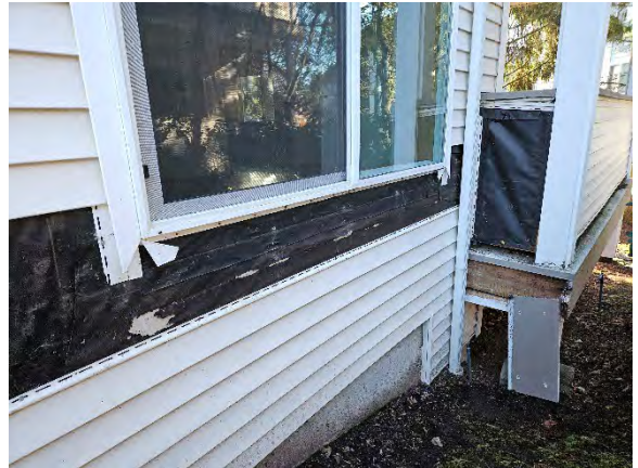
Photo 1.2: Opening following cladding removal.
