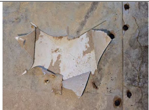
Photo 16.6: Water damaged gypsum sheathing, paper facing, and fasteners.
