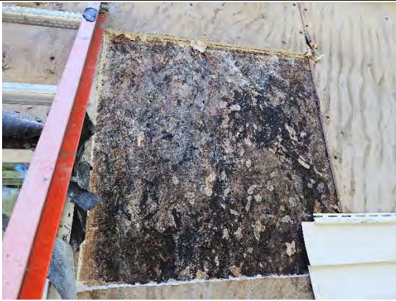
Photo 16.9: Water damaged OSB sheathing.
