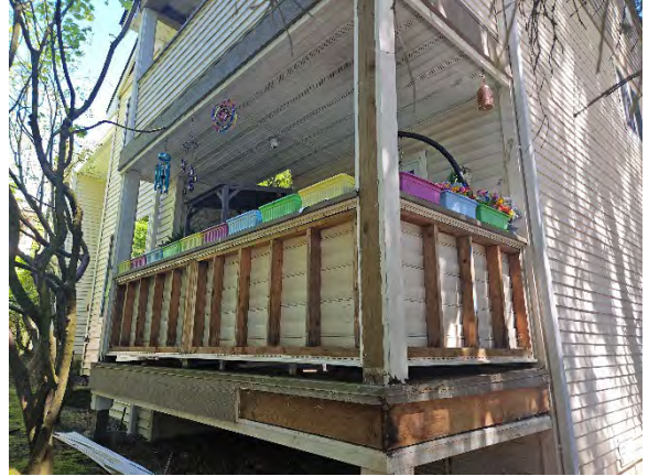
Photo 10.2: Opening following cladding removal.
