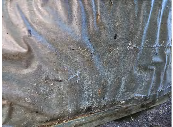
Photo 5.4: Water damaged WRB.
