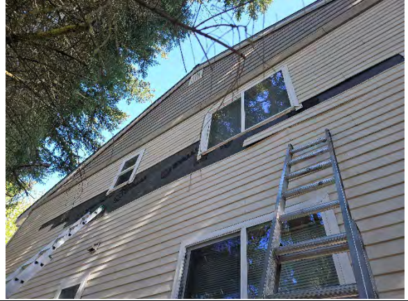
Photo 4.2: Opening following cladding removal.
