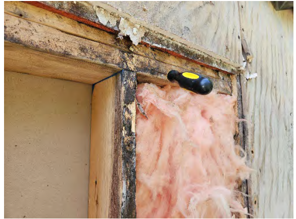
Photo 16.14: Water damaged framing.
