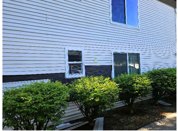
Photo 1.2: Opening following cladding removal.
