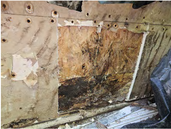
Photo 5.7: Water damaged OSB sheathing.
