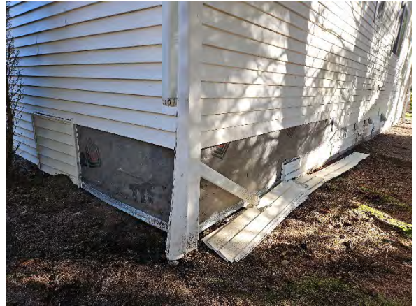
Photo 3.2: Opening following cladding removal.
