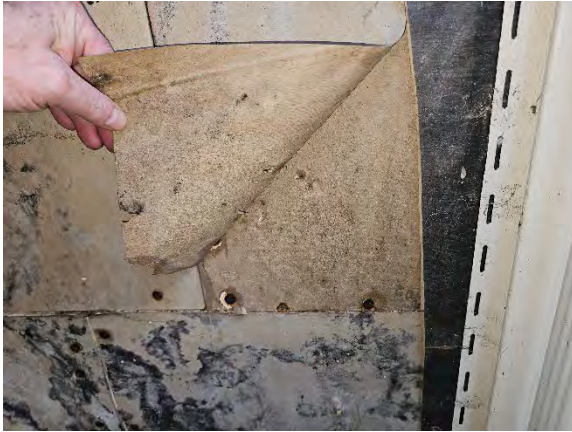
Photo 12.3: Water damaged gypsum sheathing, paper facing, fasteners, and core.
