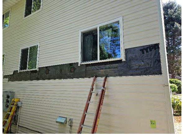
Photo 14.2: Opening following cladding removal.
