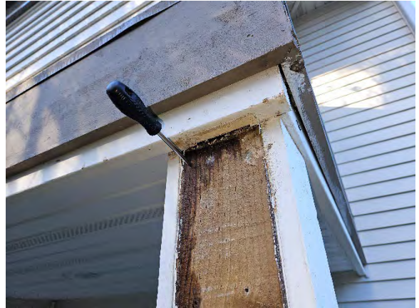
Photo 2.4: Water damaged deck column.
