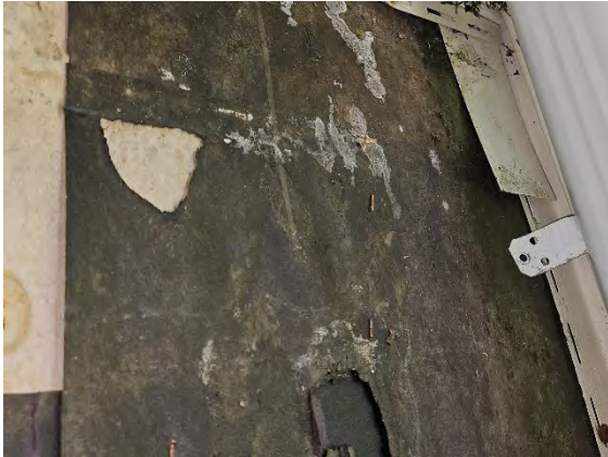
Photo 9.3: Water damaged WRB.
