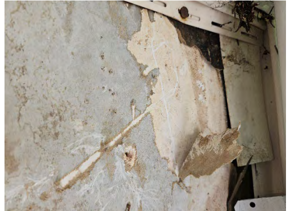
Photo 9.4: Water damaged gypsum sheathing, paper facing, fasteners, and core.
