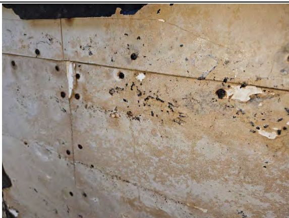
Photo 8.5: Water damaged gypsum sheathing, paper facing, fasteners, and core.
