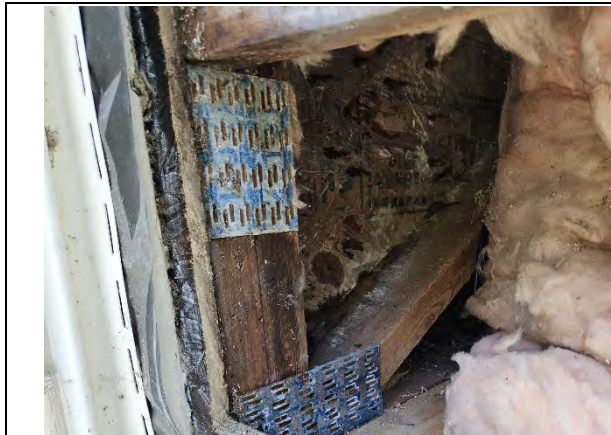
Photo 15.13: Water damaged framing.
