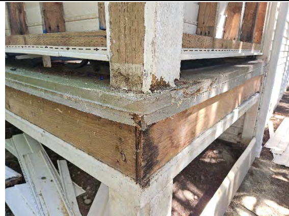
Photo 10.3: Water damaged deck framing.
