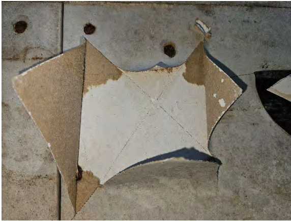
Photo 3.7: Water damaged gypsum sheathing, paper facing, and fasteners.
