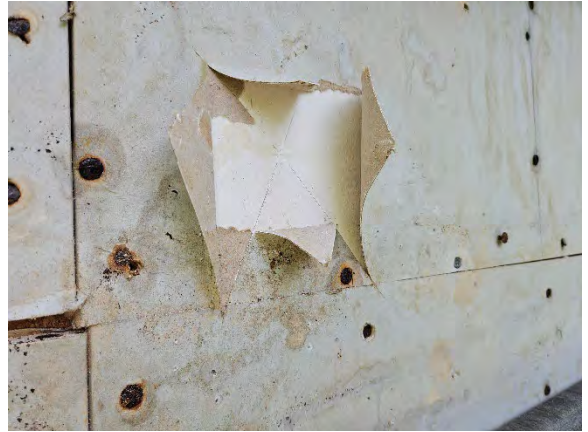
Photo 14.4: Water damaged gypsum sheathing, paper facing, and fasteners.
