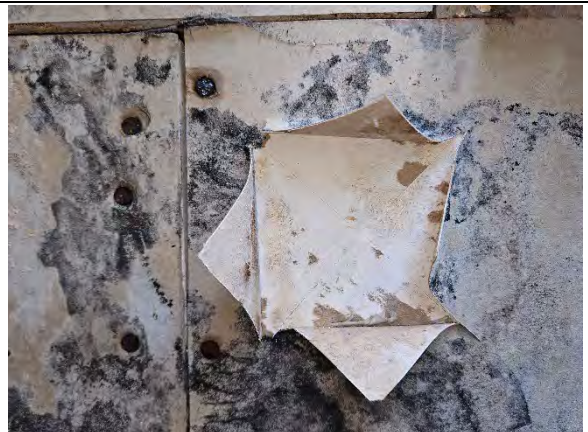
Photo 12.6: Water damaged gypsum sheathing, paper facing, and fasteners.
