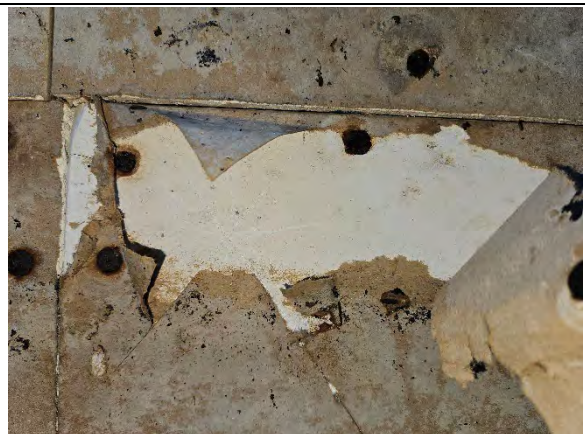
Photo 8.6: Water damaged gypsum sheathing, paper facing, fasteners, and core.
