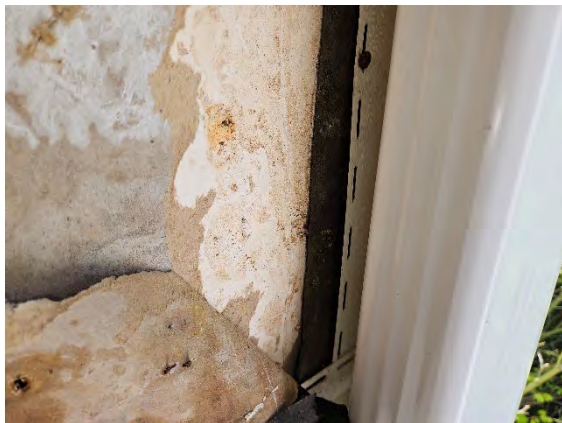
Photo 9.5: Water damaged gypsum sheathing, paper facing, fasteners, and core.
