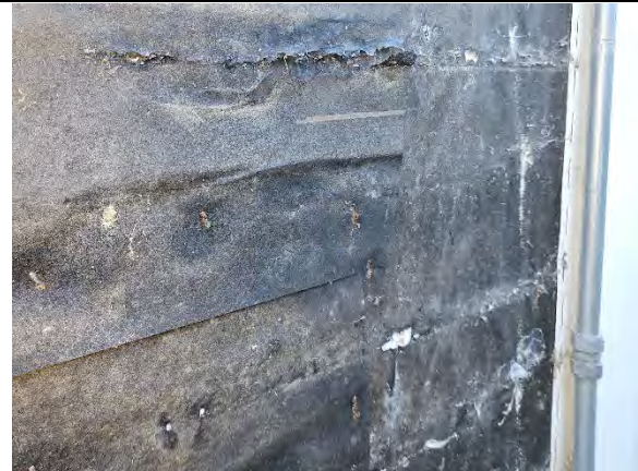
Photo 1.4: Water damaged WRB.
