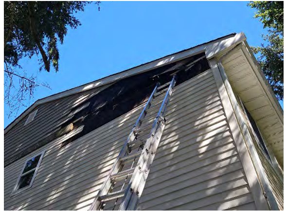
Photo 3.2: Opening following cladding removal.
