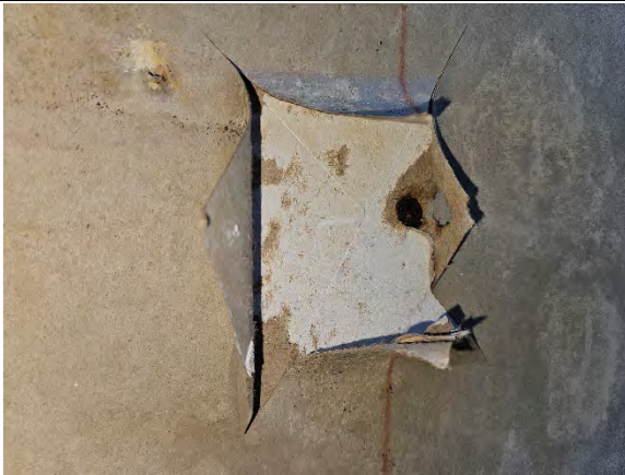
Photo 6.3: Water damaged gypsum sheathing, paper facing, and fasteners.
