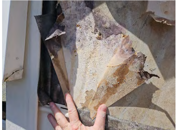
Photo 13.4: Water damaged gypsum sheathing, paper facing, fasteners, and core.
