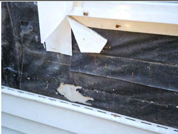
Photo 1.3: Water damaged WRB.
