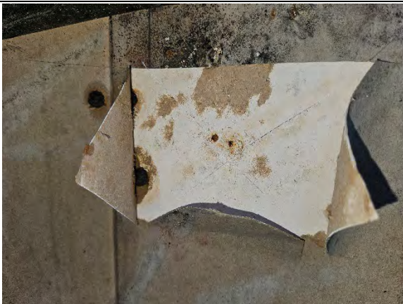
Photo 12.5: Water damaged gypsum sheathing, paper facing, fasteners, and core.
