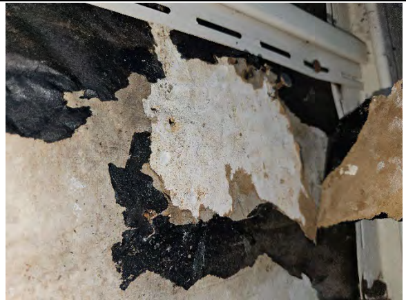
Photo 3.4: Water damaged WRB.
