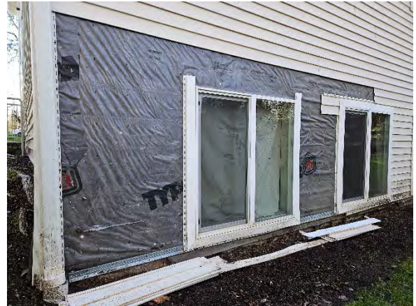
Photo 6.2: Opening following cladding removal.
