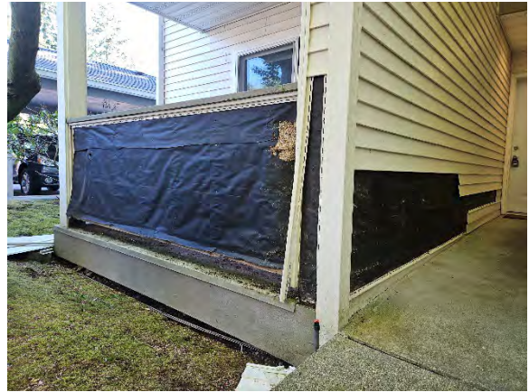
Photo 2.2: Opening following cladding removal.
