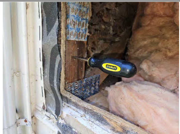
Photo 15.14: Water damaged framing.
