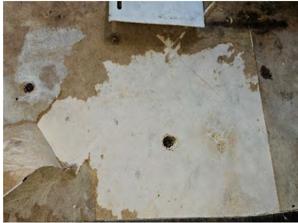
Photo 5.3: Water damaged gypsum sheathing, paper facing, and fasteners.
