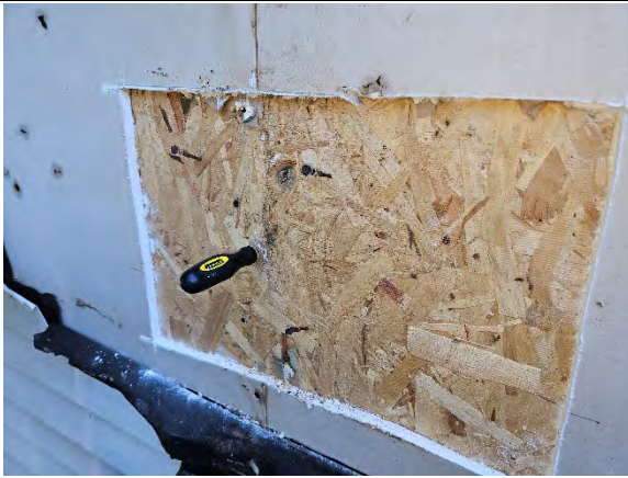
Photo 1.9: Water damaged OSB sheathing.
