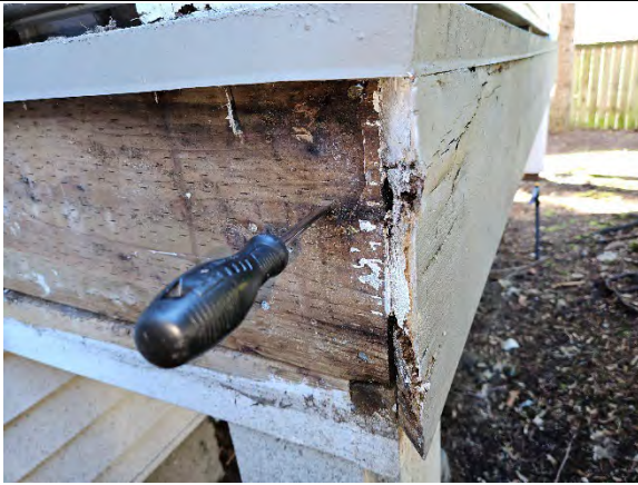
Photo 1.9: Water damaged deck framing.
