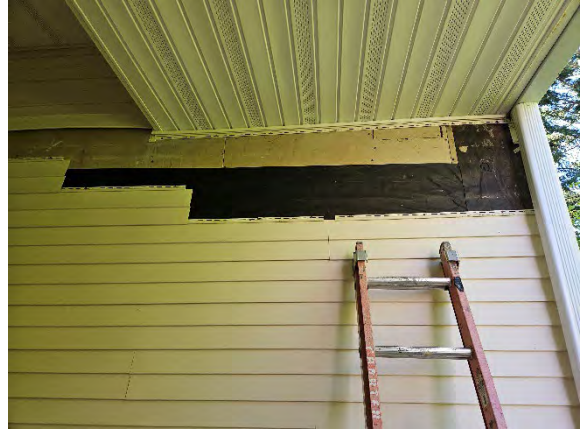
Photo 9.2: Opening following cladding removal.
