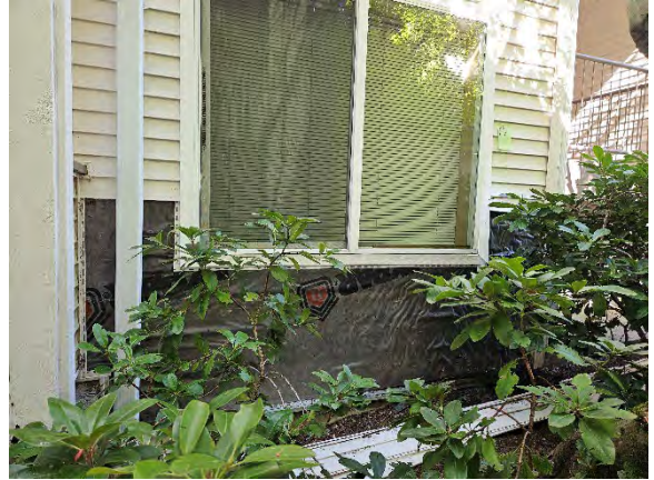
Photo 5.2: Opening following cladding removal.
