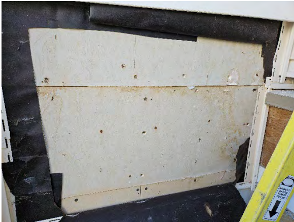
Photo 4.3: Opening following WRB removal.
