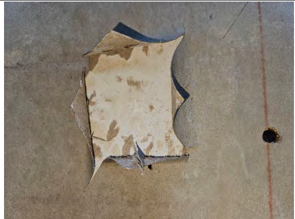
Photo 6.4: Water damaged gypsum sheathing, paper facing, and fasteners.
