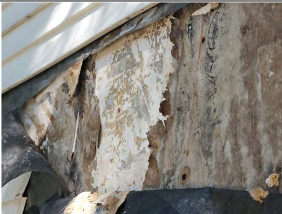
Photo 4.5: Water damaged gypsum sheathing, paper facing, fasteners, and core.
