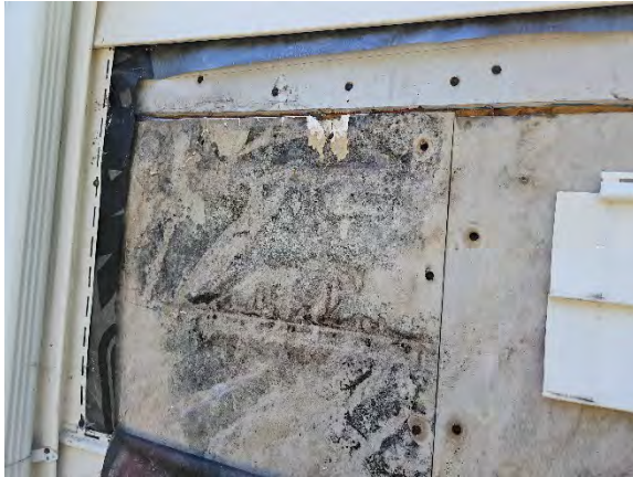
Photo 15.3: Water damaged gypsum sheathing, paper facing, fasteners, and core.
