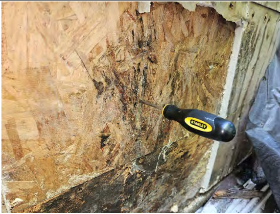
Photo 5.9: Water damaged OSB sheathing.
