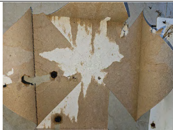
Photo 6.5: Water damaged gypsum sheathing, paper facing, and fasteners.
