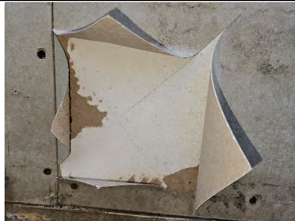
Photo 6.3: Water damaged gypsum sheathing, paper facing, and fasteners.
