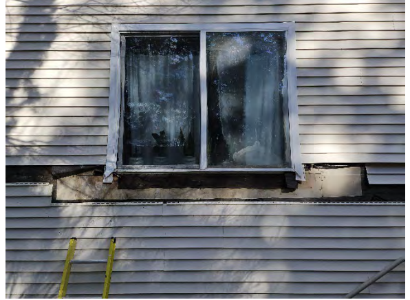
Photo 5.2: Opening following cladding removal.
