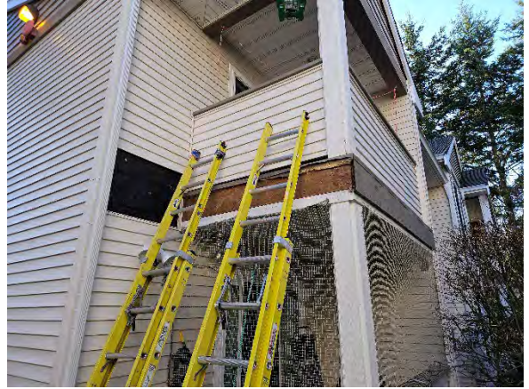
Photo 4.2: Opening following cladding removal.
