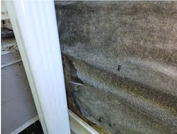
Photo 5.3: Water damaged WRB.
