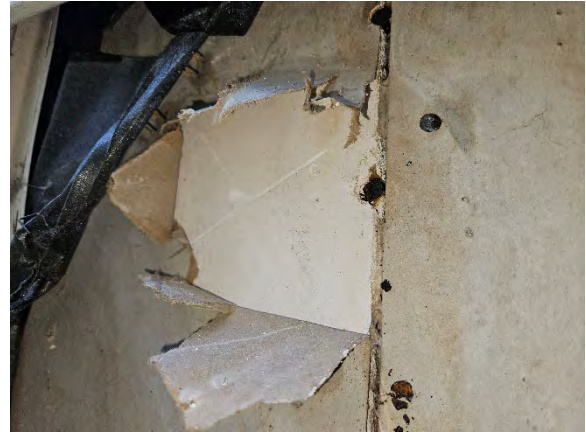
Photo 11.4: Water damaged gypsum sheathing, paper facing, fasteners, and core.
