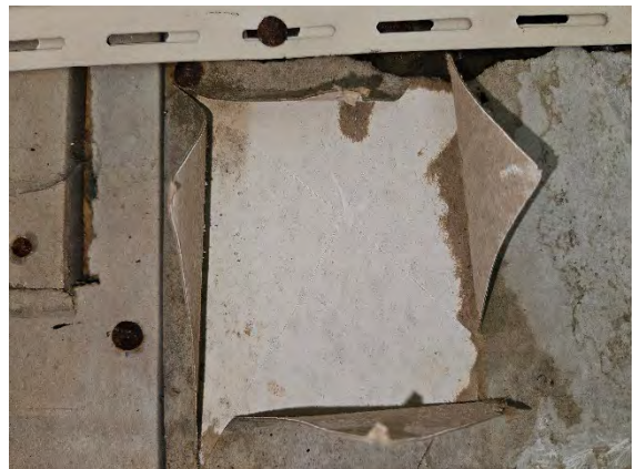
Photo 9.6: Water damaged gypsum sheathing, paper facing, and fasteners.
